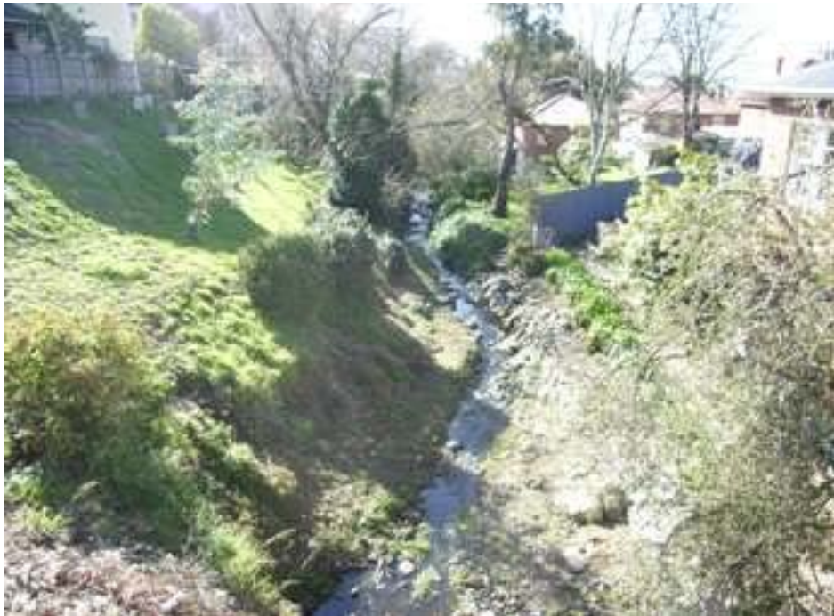
Figure 4: Some areas of the Rivulet may pose problems in terms of property impact and construction
