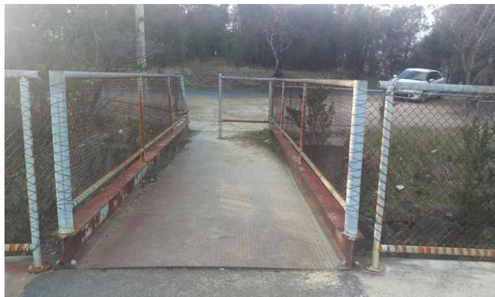
Existing entry to Eastern Reservoir - traffic management and access to this area to be improved
