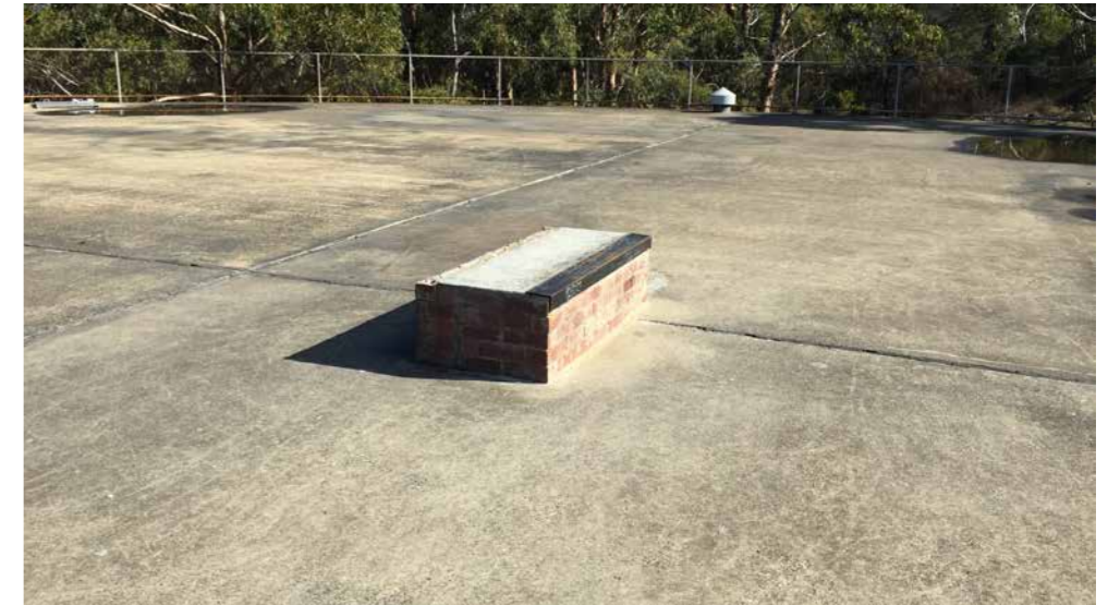
Skatable elements installed on water tank by users, shows keen interest
