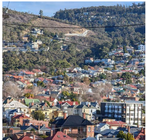
View of Sandy Bay from Short Beach towards Southern Outlet both areas prone to natural hazards.
