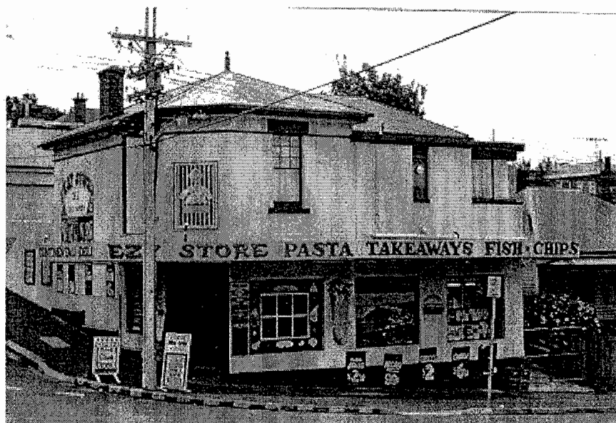
Figure 4.14 Corner shop at the intersection of Hill and Warwick Streets. It has framed the corner of this major intersection since 1916.
