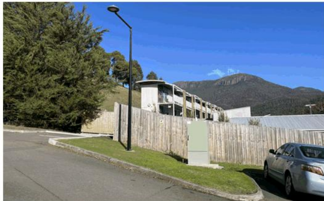
Figure 3: The previous temporary housing development as viewed from the council carpark adjoining the subject site.
