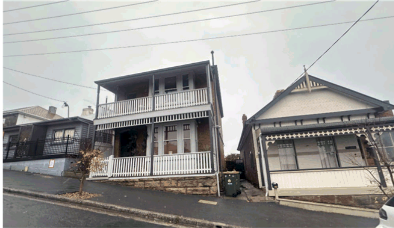
Figure 3: Streetscape view (subject site on the left)
