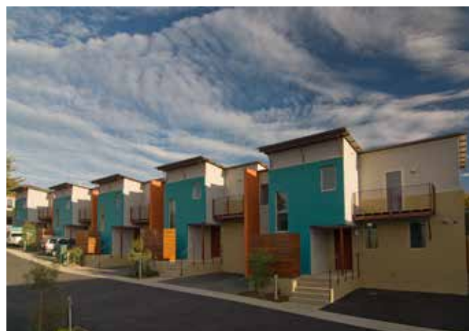
Terrace housing in Hobart designed by Morrison Breytenbach Architects.
