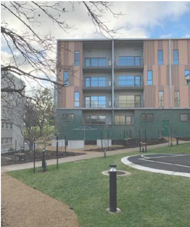
Queens Walk affordable and social housing designed by Cumulus Architects for Housing Choices.
