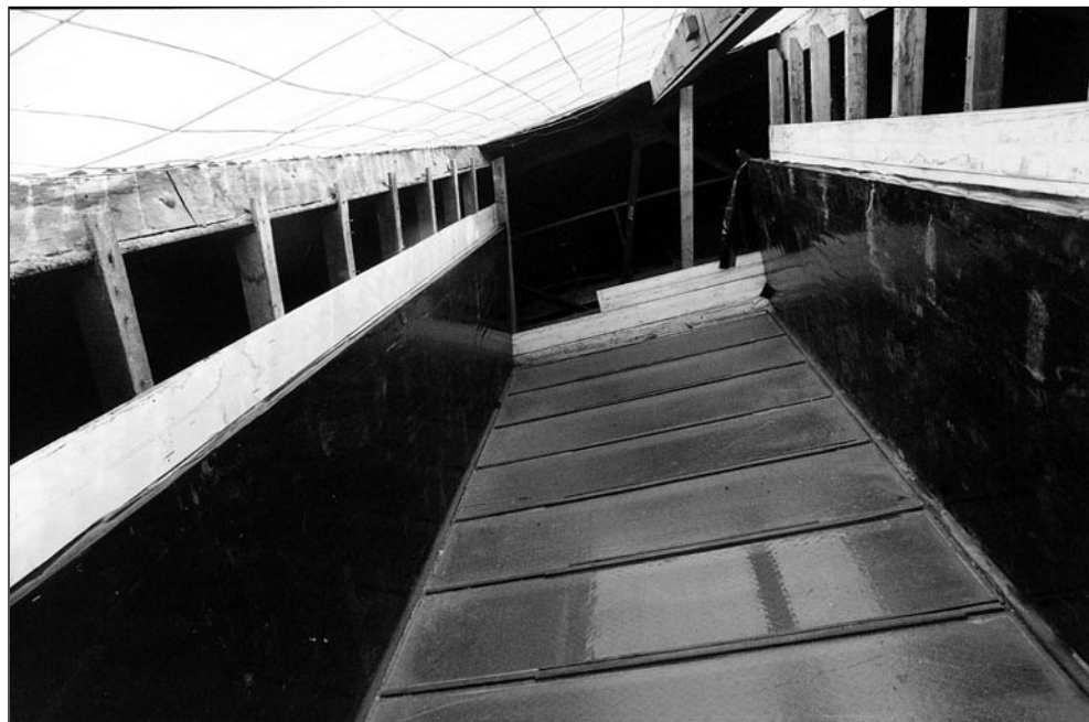
Figure 77. Auditorium skylight showing black plastic covered shutters.
