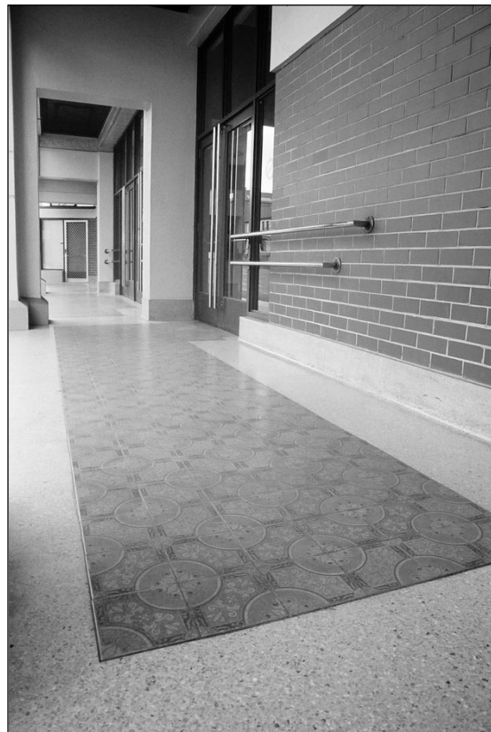
Figure 50. Tiles and terrazzo laid outside foyer in 1975 refurbishment. The wall on the right previously contained shop front windows.
