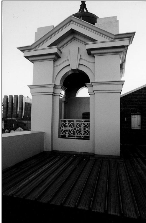
Figure 53. Rooftop tower on Market Place side of building..
