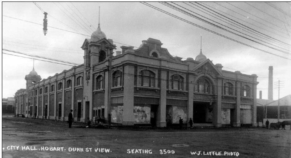
Figure 7. The City Hall and Market Place nearing completion. Note the twin doorways next to the shopfront on Market Place to the ticket office and upstairs rooms (AOT — NS 526/11).
