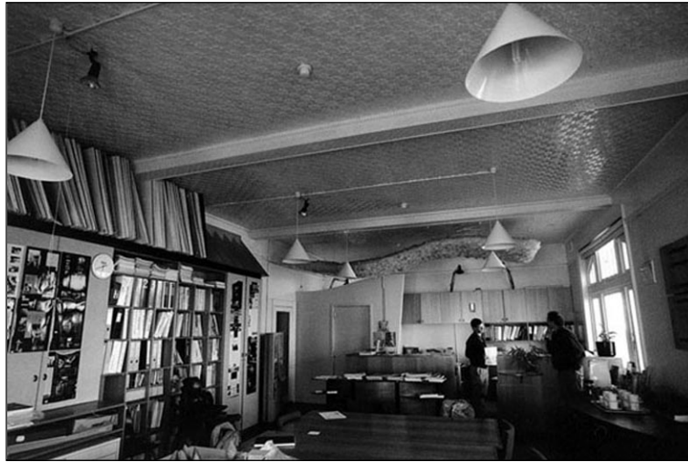
Figure 59. Interior of the RAIA office. Note the pressed metal ceiling and the bookcase on the left concealing the original door to the auditorium gallery.
