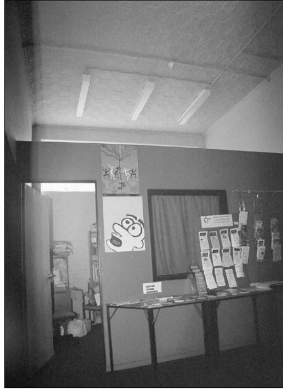
Figure 86. YouthArc office at the former 44 Collins Street shop with partitioned wall, strip lighting and conduits laid over pressed metal ceiling.
