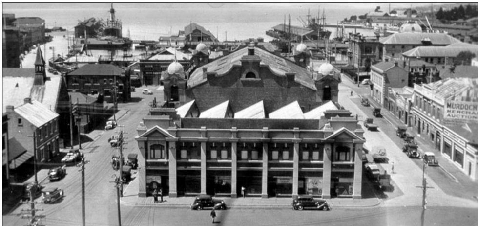
Figure 37. Collins Street end of the City Hall in the 1930s. Note the location of the doors and windows to the shops. Note also the setting and compare with figures 5 and 87. (AOT — NS869/409).
