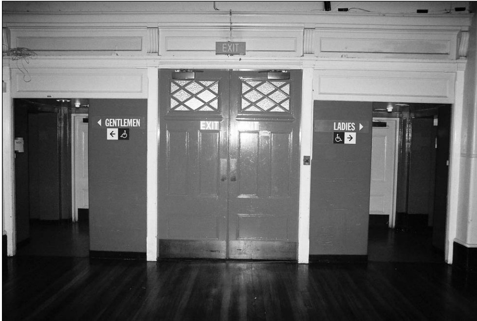
Figure 65. Doors linking foyer to auditorium and between auditorium and toilets. Prior to 1974 there were three double doors between the foyer and the auditorium.
