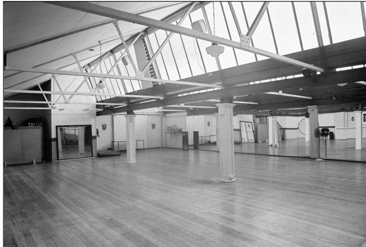
Figure 88. Dance studio showing timber floor, sawtooth roof and doors to upper backstage area in background.
