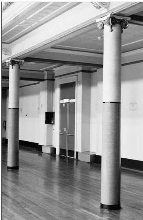
Figure 66. Partially vinyl covered columns on Market Place side of auditorium.
