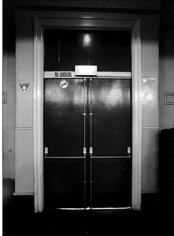
Figure 67. Exit doors to Market Place covered with acoustic material.
