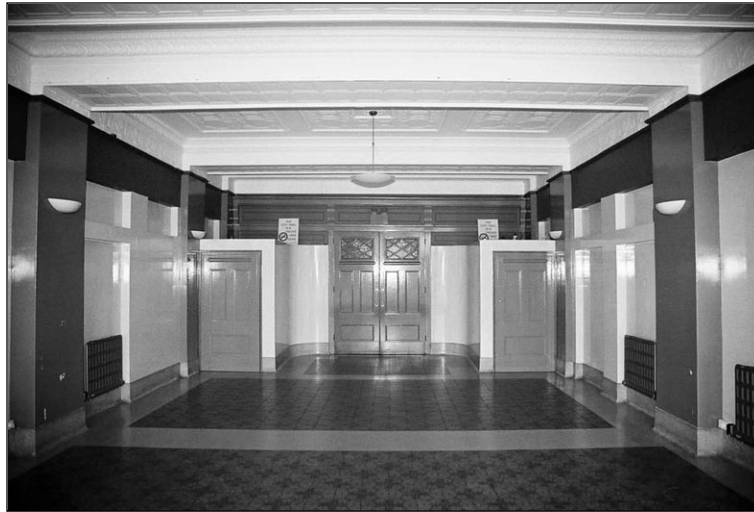
Figure 54. Foyer looking towards auditorium doors in 2001. Note tiled floors and pressed metal ceiling.
