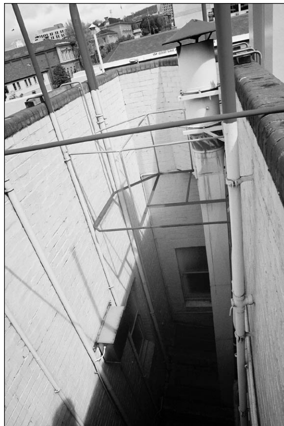
Figure 52. Lightwell above foyer showing structure to support 63 Macquarie Street exhaust fan.
