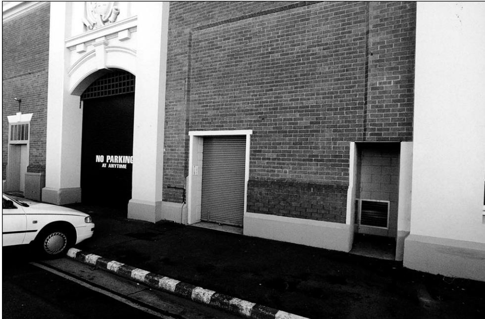
Figure 47. Market door and door to electrical substation (centre) on Market Place.
