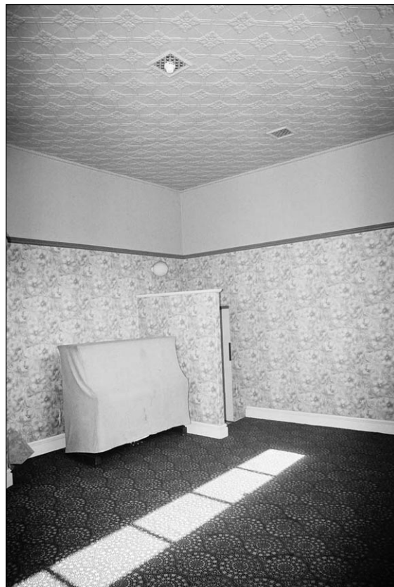
Figure 57. VIP room showing original pressed metal ceiling, 1970s era wallpaper and carpet and piano. The door at the rear is to the toilet.
