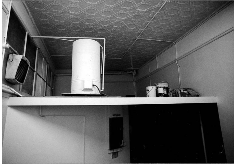
Figure 58. Space adjacent to foyer female toilets showing false ceiling and original pressed metal ceiling.
