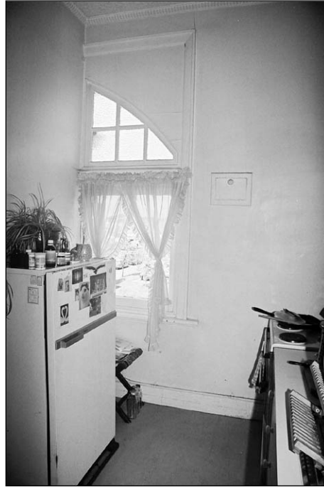
Figure 60. Caretaker's flat kitchen. Note the vent door and the truncated window (cf façade).
