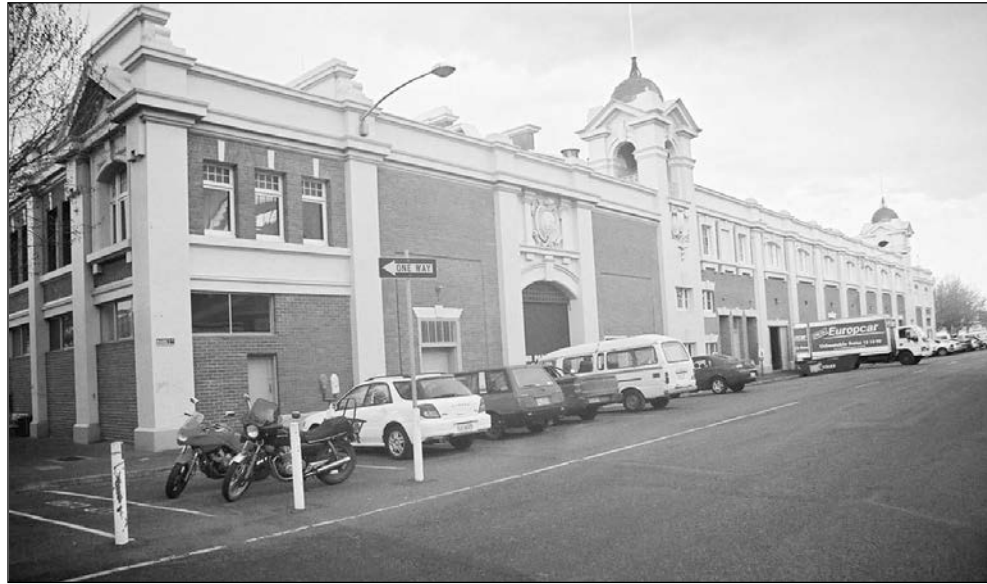
Figure 45. Market Place façade.
