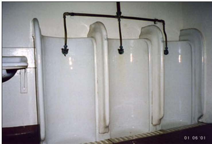
Figure 74. Original urinals in gallery toilets. Similar urinals remain in the foyer men's toilets.
