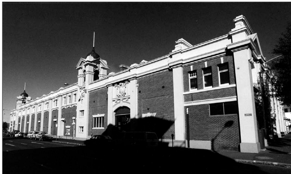
Figure 46. Campbell Street façade.
