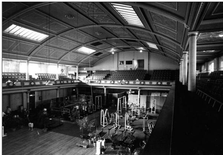
Figure 64. Interior of Auditorium from gallery looking towards rear. Note ornate pressed metal ceilings, skylights and projection box windows at rear. cf figure 12 showing just one projection box window.
