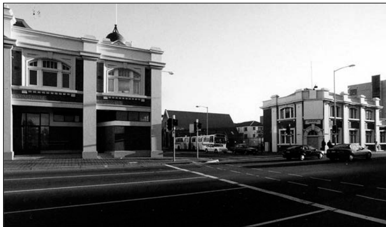
Figure 90. Macquarie/Campbell Streets streetscape showing former MTT offices and St David's Church.
