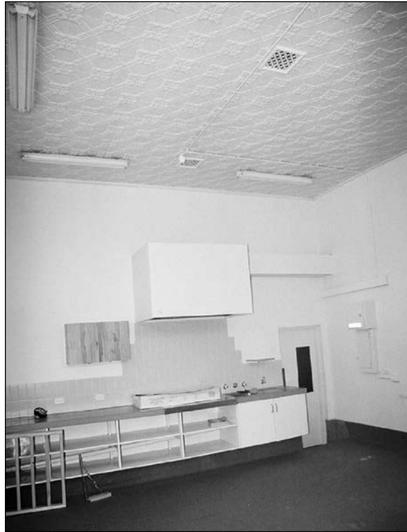
Figure 56. Interior of 63 Macquarie Street showing original pressed metal ceiling and 1970s kitchen bench and tiling.
