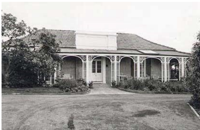
Beaulieu built in the late 1820s is an early Colonial stone home with fine Regency details. Photograph c.1940s. (Australian Heritage Database)
