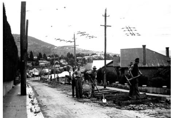
Workers digging on Proctors Road, c.1940s. (AOT: NS1029 169)
