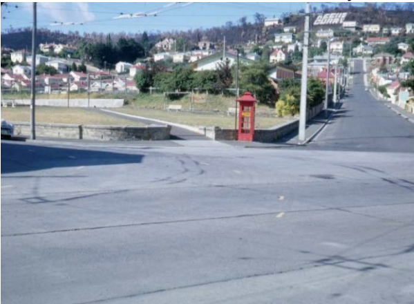
Intersection of Wentworth and Washington Street after 1967 bushfires (AOT NS2297 151)
