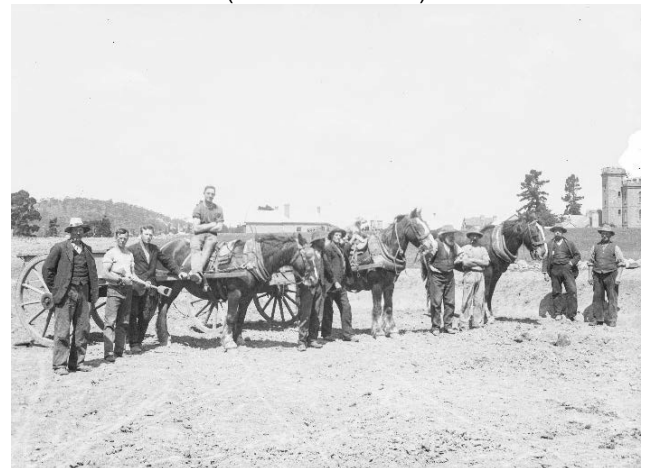
Road construction team on New Town Road near Tower Road c.1900 (AOT NS392-1-162)
