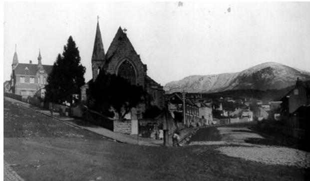
Intersection of Goulburn St & Forest Rd - St John the Baptist church in foreground and Mt Wellington in the background c.1920 (ATO PH30-1-6992)
