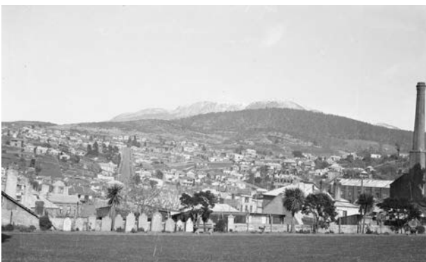
Trinity Hill burial ground before demolition (ATO NS1231122)
