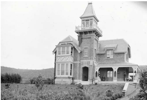
100 King Street 'Selborne' designed by architect Henry Hunter c. 1880s. (AOT: NS1013 1540)
