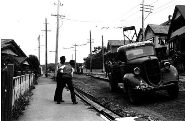
Workers laying drains in Proctors Road, c.1940s. (AOT: NS1029 168)
