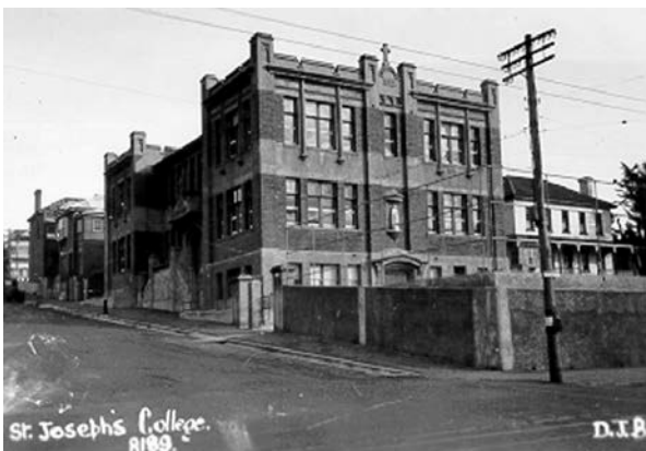
External view of St Joseph's College on the corner of Molle and Macquarie streets (AOT: PH30-1-4637)
