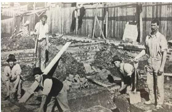
Worker laying the foundations of a new house on Lord Street c.1919. (Lord, G. 1998.)
