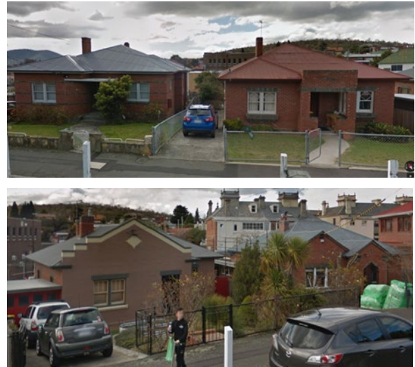
Figure E16: Examples of the housing to be included in the precinct.
