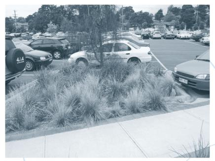
Bioretention planters in a large car park. Car park runoff is directed into garden beds with underdrainage (and overflow points) to clean and slow runoff. Runoff enters garden bed via breaks in the curb (see bottom right of garden).
