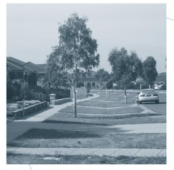
Residential swale drainage at Lynbrook Estate, Melbourne. Shallow batter slopes on the drain allow driveway crossovers without the need for culverts. Swale width and regular drains delivering flow to a piped underground stormwater system mean that flows are rarely deeper than grass height.
