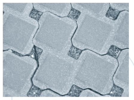
*Close up view of permeable paving. Gaps in pavers are filled with 'clean' gravel allowing water to infiltrate to the ground below.*
