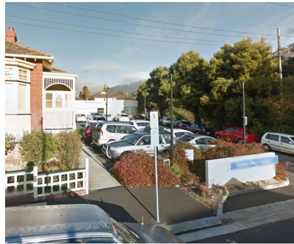
Figure E2: Photo of the carpark to be removed from the precinct.
