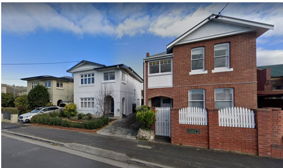
Figure E20: 40, 42 and 44 Regent Street
