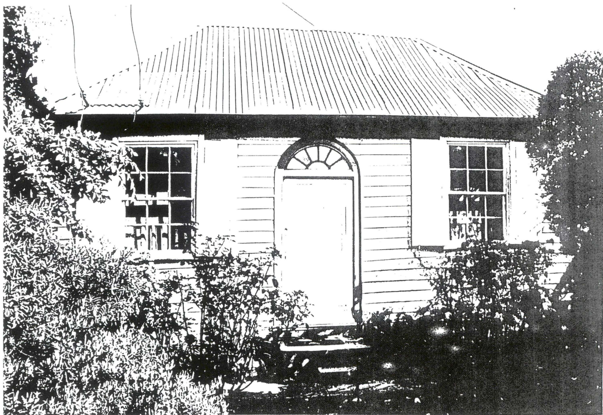
"Generally regarded as being the oldest timber structure in Hobart", this weatherboard house at 225 Collins Street is possibly the sole survivor of its type in the study area (Bolt, p. 192)
