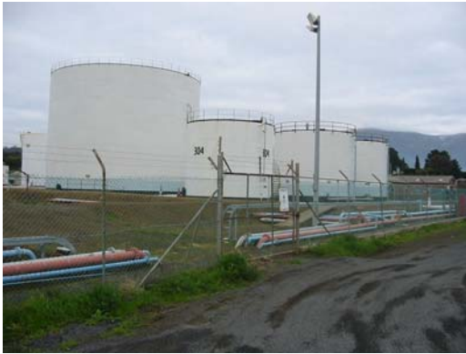
Oil Storage Tanks (Site 9)
