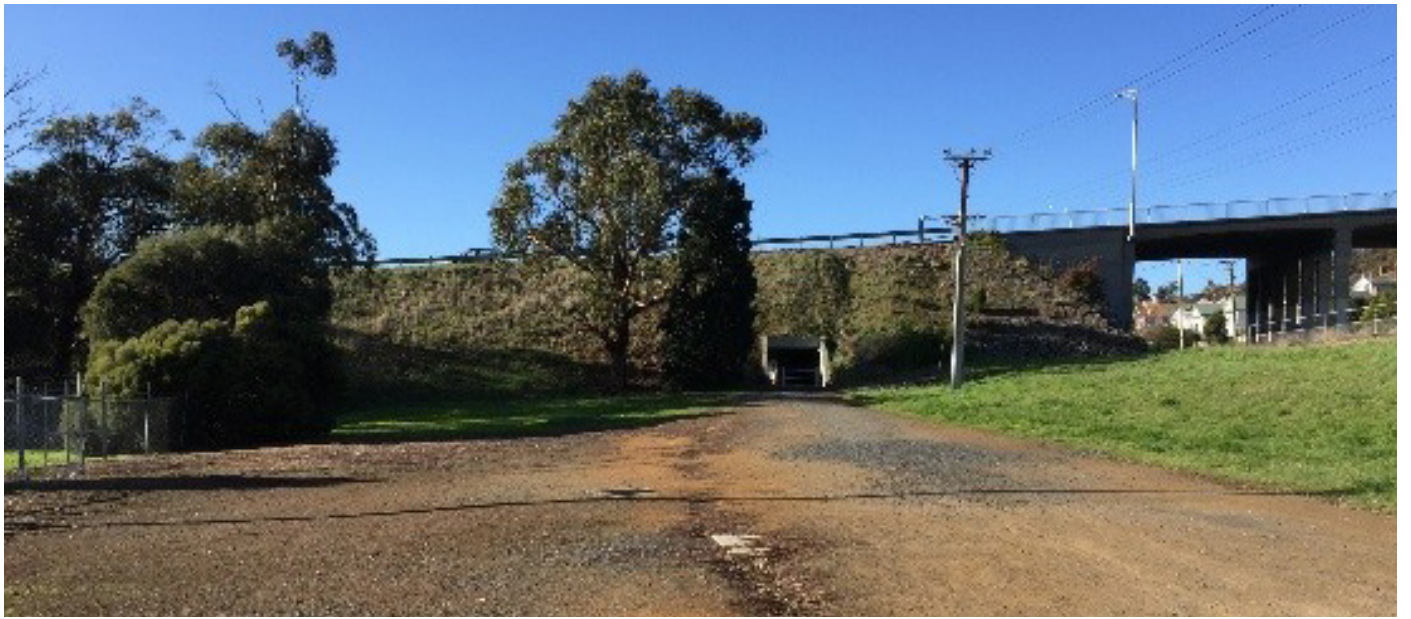
Pedestrian subway under Brooker Highway at Bell Street
