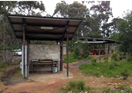
Lightweight timber structures
