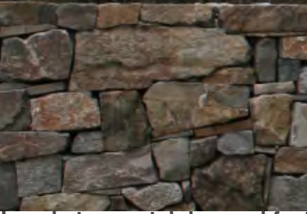
Local stone retaining and feature walls
