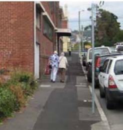
Worn-out patchwork pavement does not leave the impression of high quality footpaths. *Collins Street*
