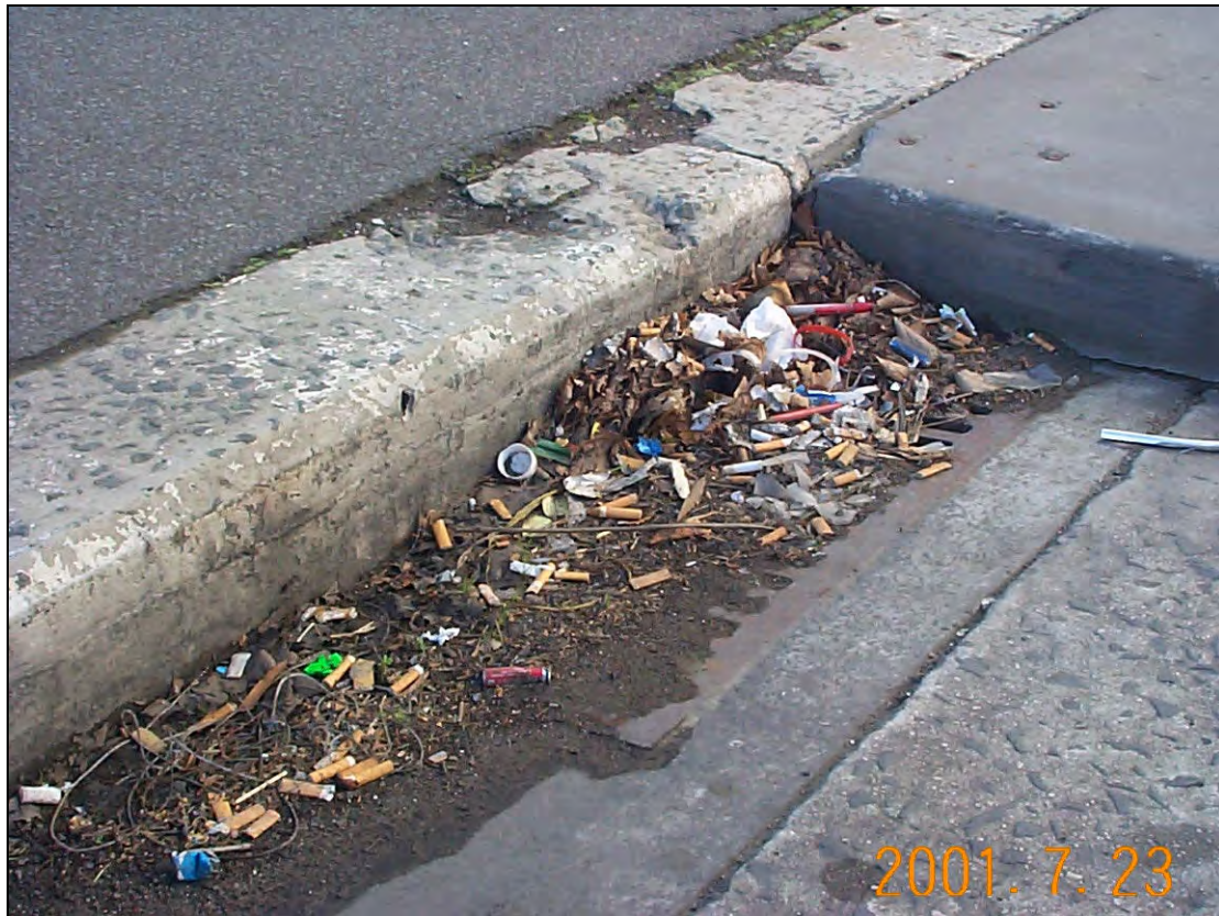
Plate 5.1 Litter accumulating in the streets and entering river systems via stormwater
