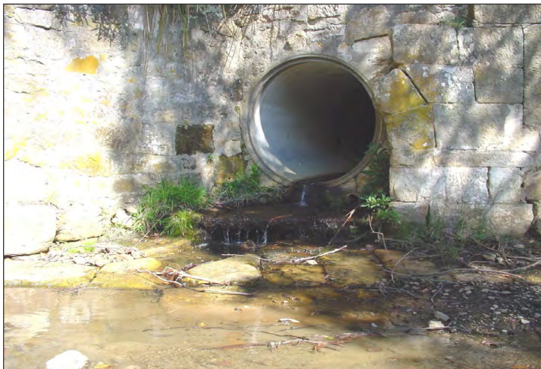
Plate 5.2 Stormwater outlets are a source of contamination from road runoff
