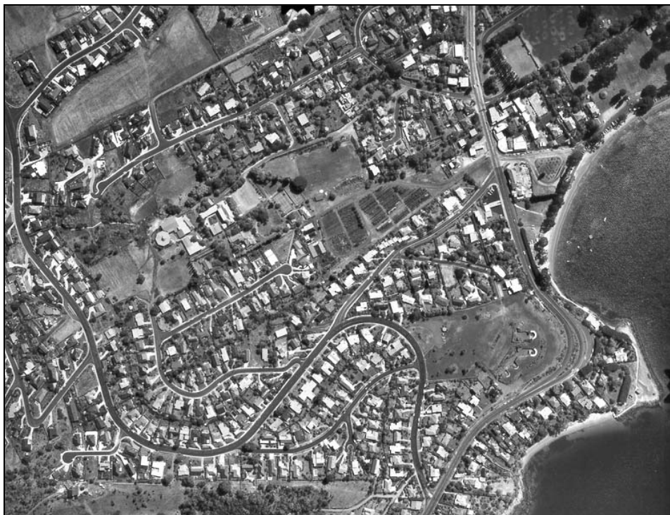
Figure 1.2 Aerial Photograph of the exposed Section of Wayne Rivulet
