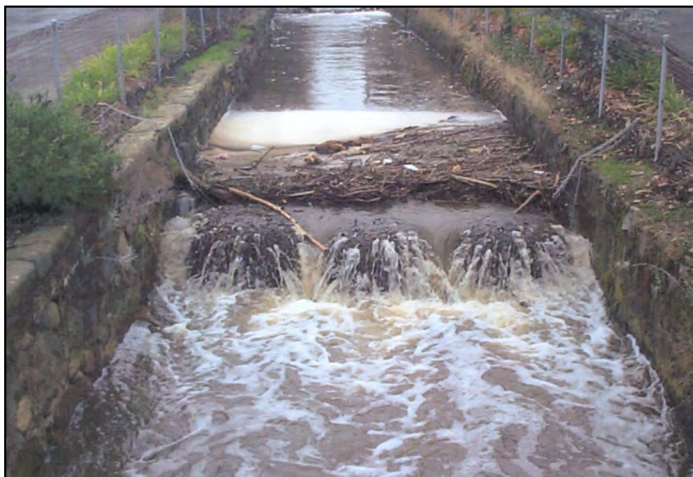
Plate 5.3 Quayle Street Litter Trap During a High Rainfall Event
