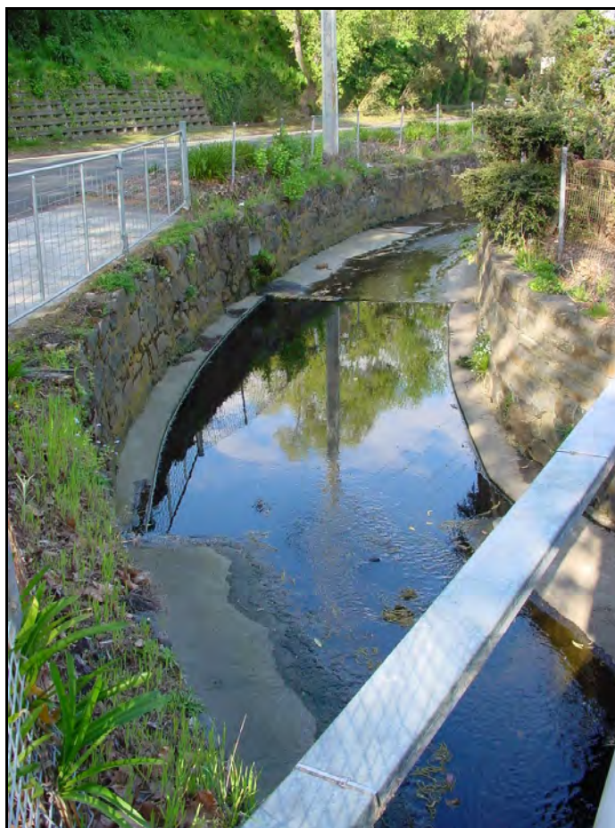
Plate 5.5 The sediment trap in Sandy Bay Rivulet
