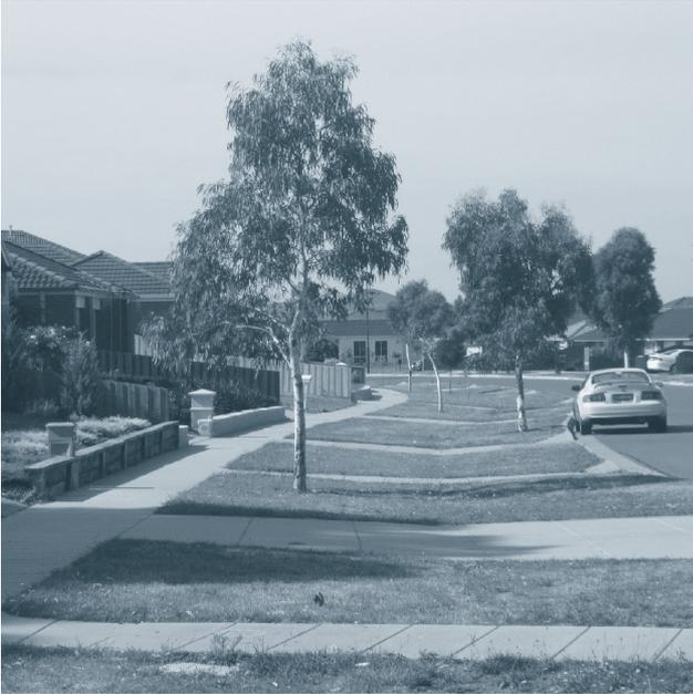
*Residential swale drainage at Lynbrook Estate, Melbourne. Shallow batter slopes on the drain allow driveway crossovers without the need for culverts. Swale width and regular drains delivering flow to a piped underground stormwater system mean that flows are rarely deeper than grass height.*
