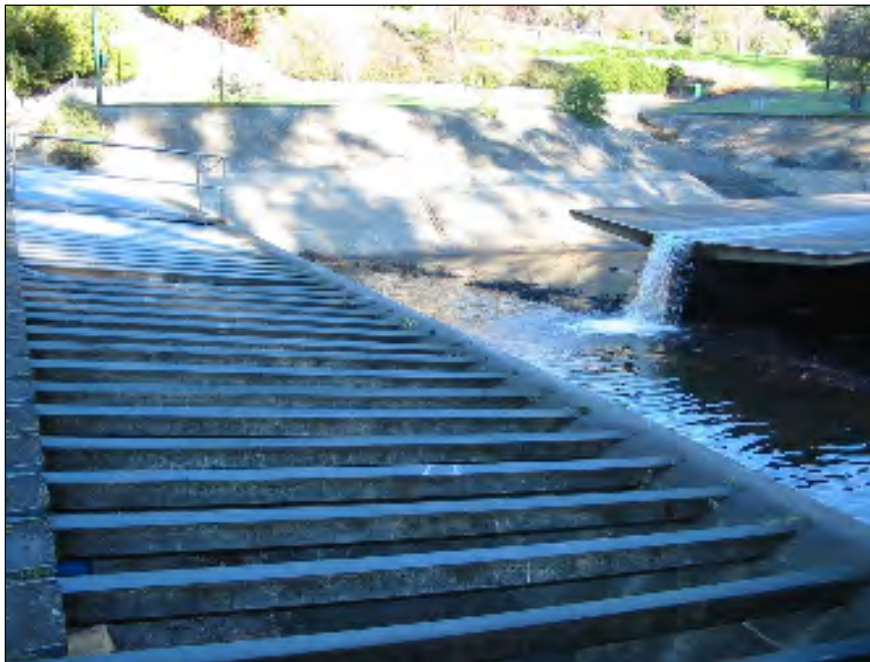
Image 6: Boulder Trap below Cascade Brewery [Source: Hobart City Council]
