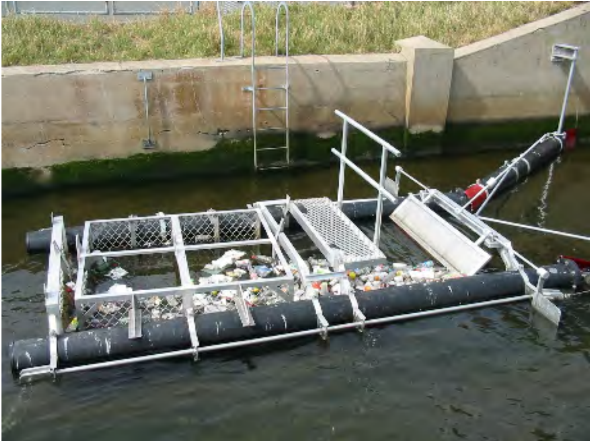
Image 11: Floating litter trap, Hobart Rivulet, Macquarie Point [Source: Hobart City Council]
