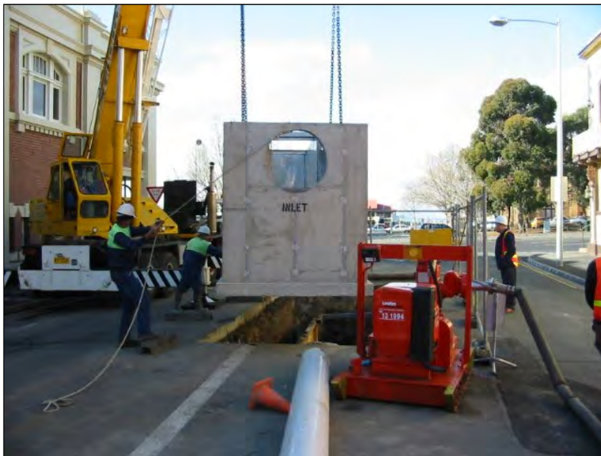
Image 10: Installation of the GPT at Market Place [Source: Hobart City Council]
