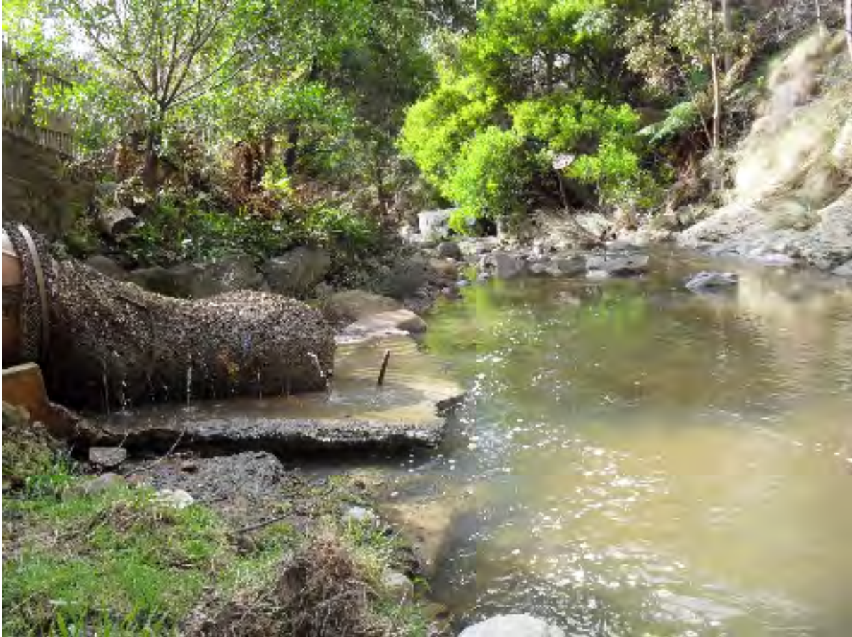
Image 12: Outpour into the Hobart Rivulet from McRobies Gully including the litter sock [Source: Hobart City Council]
