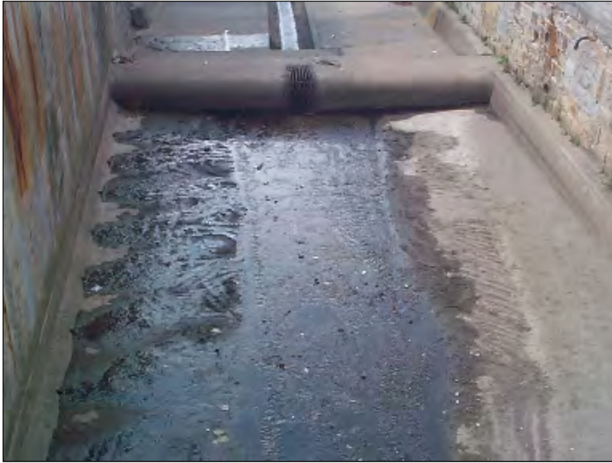
Image 7: Silt Trap after the Goulburn Catchment Outfall [Source: Hobart City Council]
