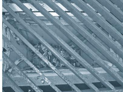
*Stormwater entry-pit trap installed in Hobart*
