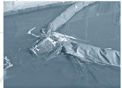
*Floating litter boom installed in Hobart*
