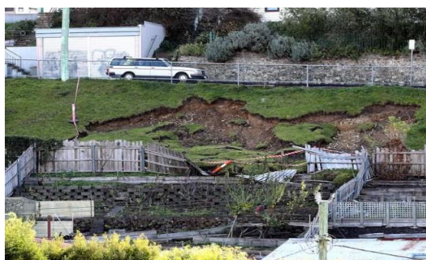
Extreme weather event in May 2018 caused significant damage to the Liverpool Street embankment and roadway.
