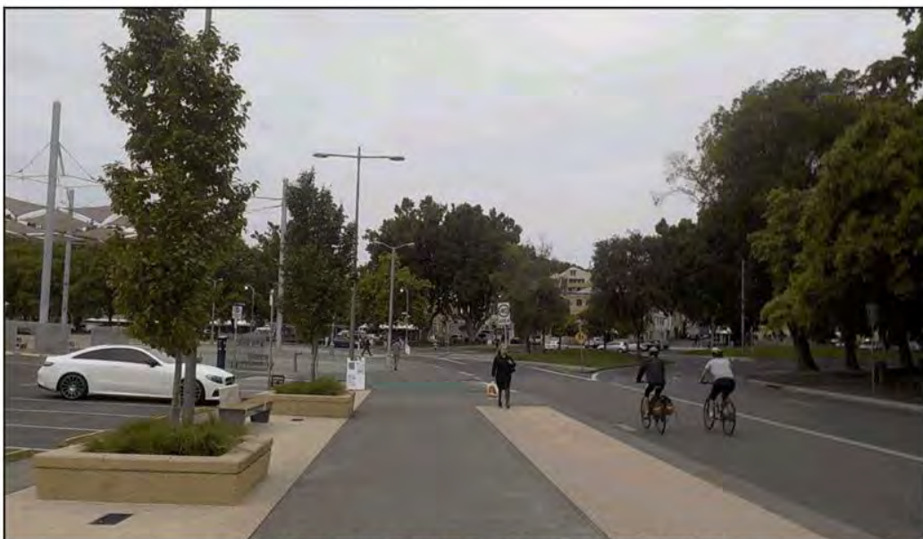
Figure 10.6 – Existing Raised Street Trees – Morrison Street
