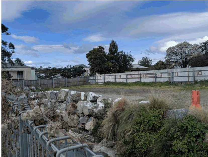
Figure 6 Northern extent of the site (Image 1). (source: E Febey)
