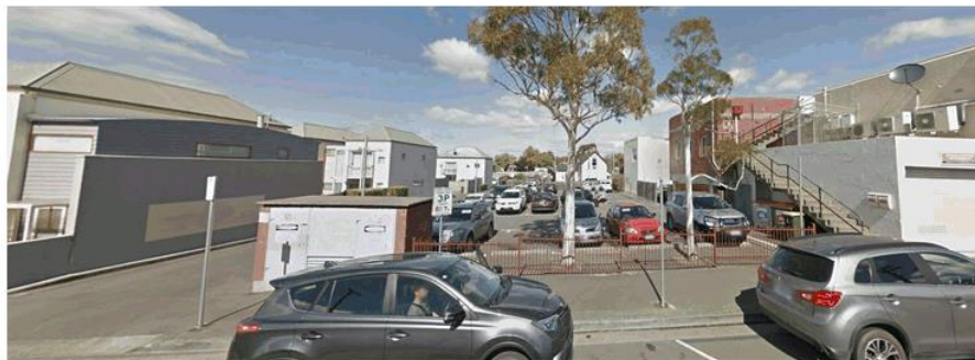
Figure 4 View of the HCC Lefroy St carpark (source: Google Maps)
