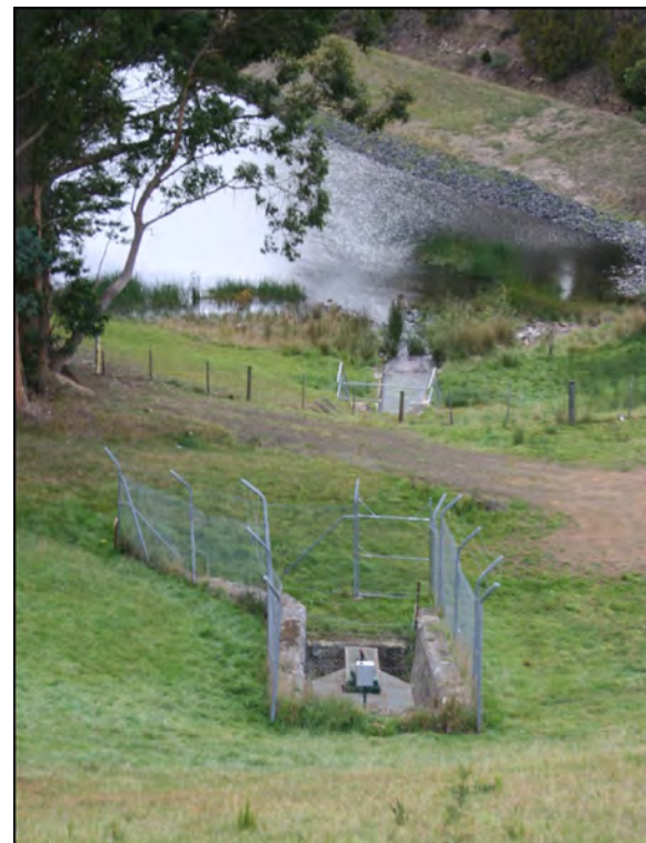
Figure 16– View of Reservoir No 1, looking down slope from Reservoir No 2 (North 2007)
