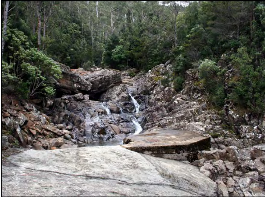
Figure 58—Contemporary view of North West Bay River Weir
