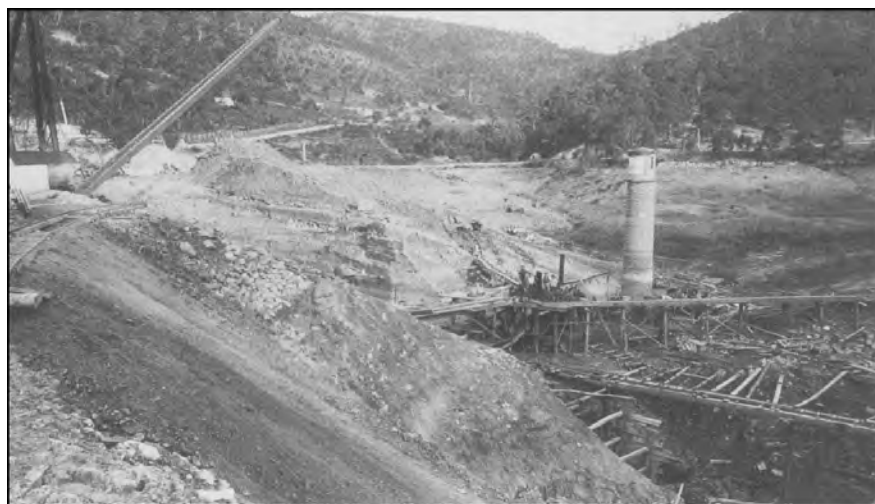
Figure 11– Reservoir No 1 under construction (Crawford and Ryan 1988: 44). Note the valve tower, which gives some impression of the depth of the reservoir.
