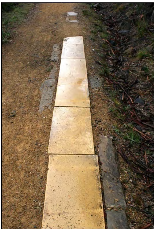
Figure 34–Inappropriate replacement covers on sandstone troughing
