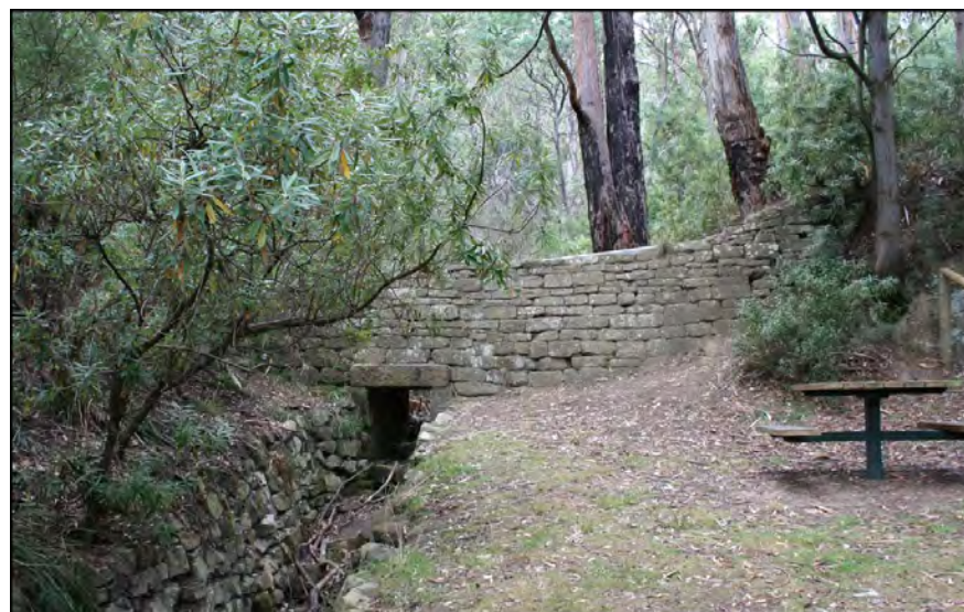
Figure 27–Dry stone walls located at the back of Regans Gully. Similar walls can be found in other locations in the Reserve.
