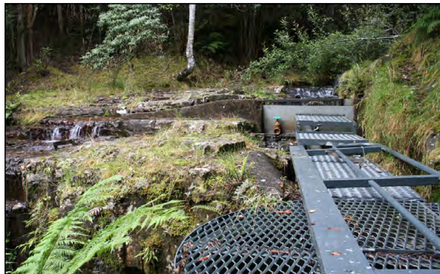
Figure 49–Intrusive equipment at Silver Falls Weir
