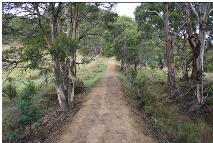
Figure 36 – The sandstone troughing near McDermott’s Saddle, facing east. In this location, the troughing is contained within a built-up earth embankment, which also serves as the pedestrian Pipeline Track route.
