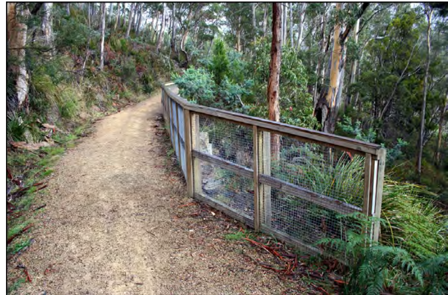
Figure 43—An example of inappropriate fencing along the pipeline. This fencing uses modern dressed timber, which is a jarring contrast to the natural and rural character of this section of the pipeline.
