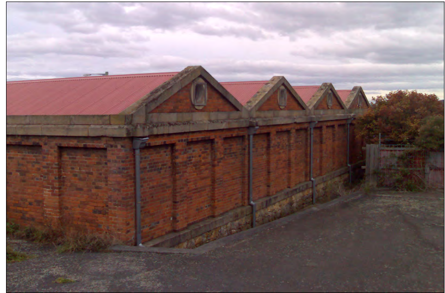
Figure 9–The Hill St service reservoir, modified but still in use. (North 2007)
