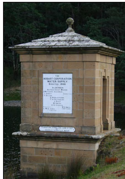
Figure 22— The Valve House for Reservoir No 2, containing the commemorative plaque for its opening in 1888. (North 2007)
