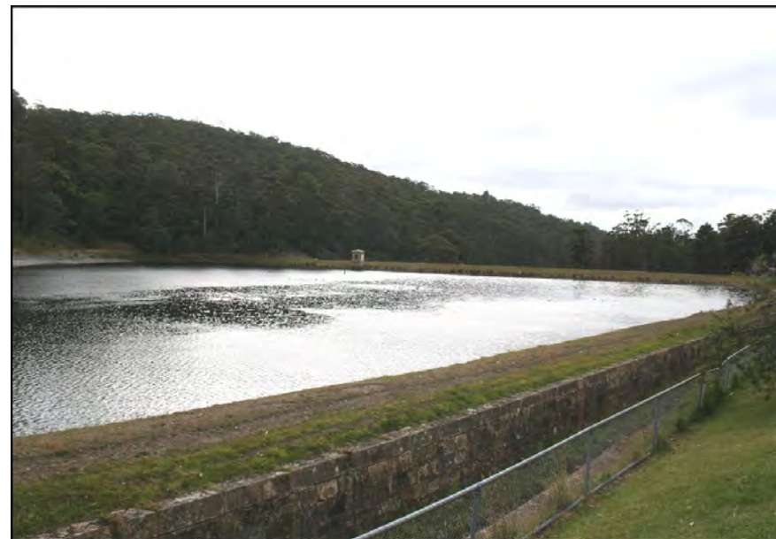
Figure 20– Reservoir No 2, with the Hard Water Channel visible alongside (North 2007)
