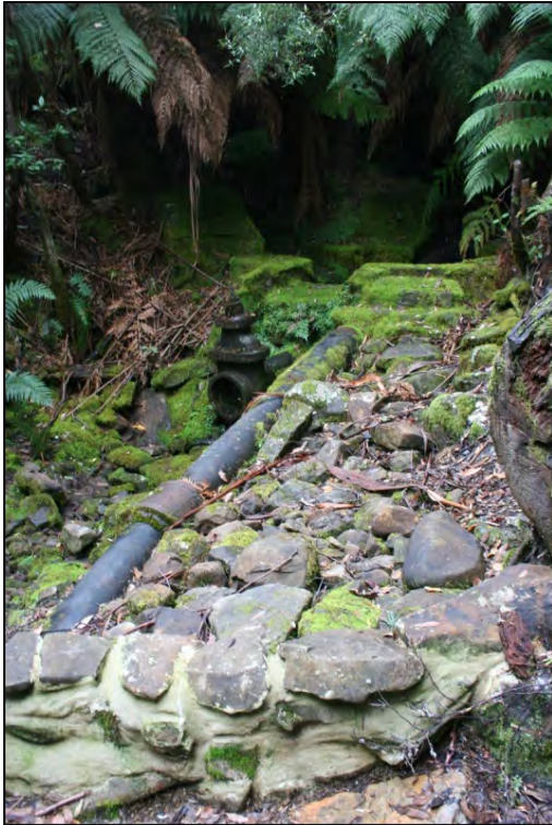
Figure 56—Intake with 20 th century supplementary stone and concrete works.
