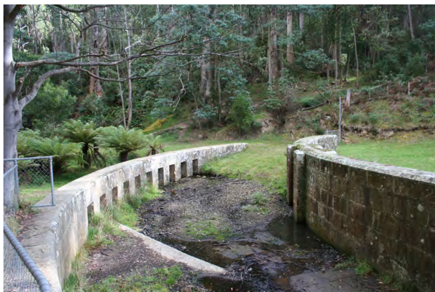
Figure 21 - The top end of the Hard Water Channel, running alongside the Upper Reservoir
