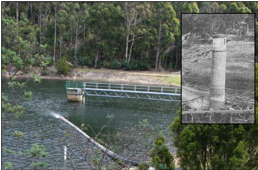
Figure 17– Reservoir No 1 Valve House.
