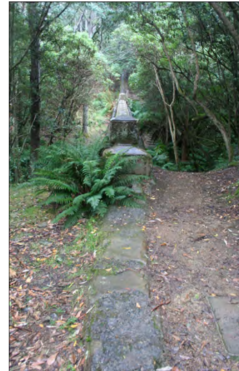
Figure 38–Aqueduct over Longhill Creek
