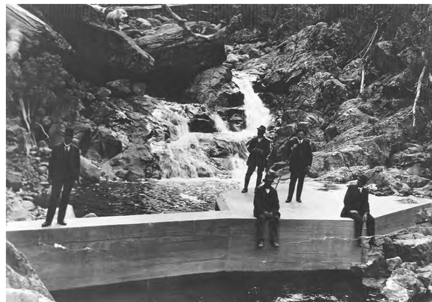
Figure 12–North West Bay River Weir shortly after construction
