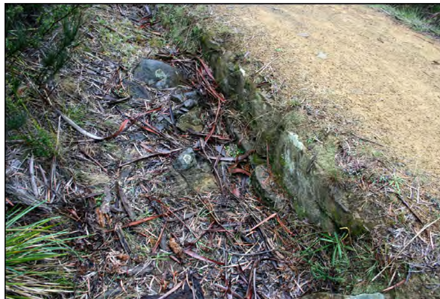
Figure 33 - The side wall of the troughing, visible in an area where the ground has been built up to form the track on top of the sandstone troughing.
