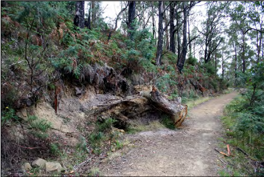
Figure 44—A tree fall across the pipeline and associated track.
