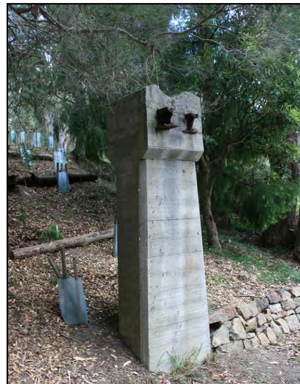
Figure 25—Concrete pipe stands
