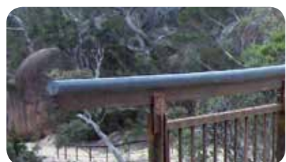
Recycled plastic handrail & mild steel components
