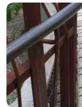
'Penetrol' on natural steel
