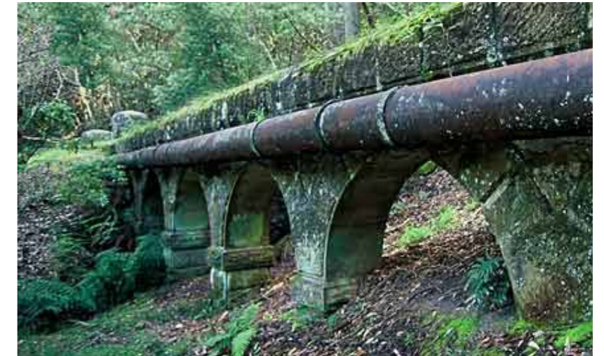
The MWSS Pipeline icon is a representation of this aqueduct which forms part of the system.
