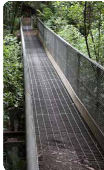
Existing Twin Bridges
