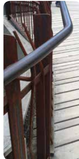
'Penetrol' on natural steel
