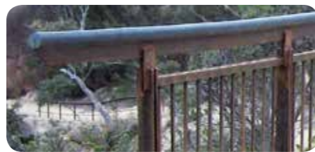
Recycled plastic handrail & mild steel components
