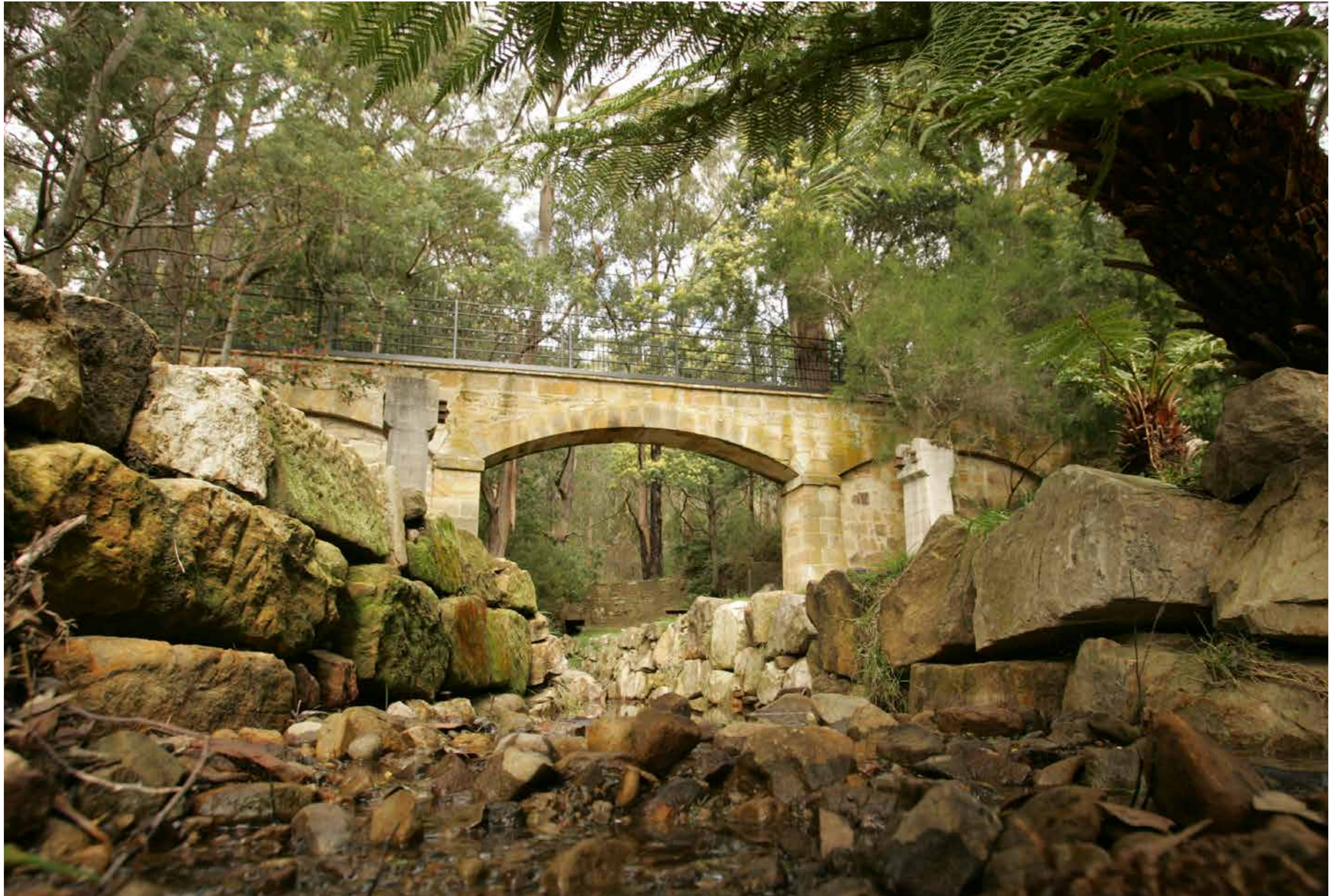
Regan's Gully Bridge, Waterworks Reserve. Photo by Eddie Safarik.
