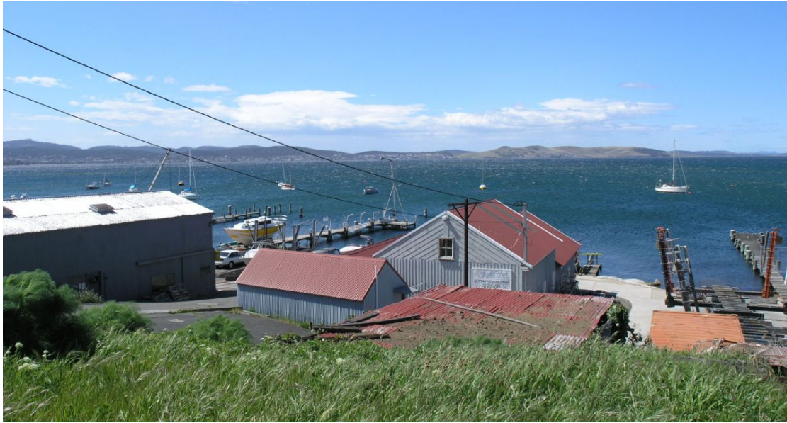
Image 3. View (V2) from embankment over Taylor Bros and Muirs slipyard areas. B13, B14, B15 and B16 are on the Taylor Bros site to the right and B12 Muirs Workshops is to the left of the image.
