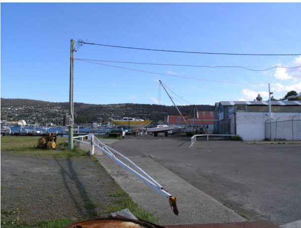
Image 31. View (V5) across the slip sites from the foreshore area in front of A4
