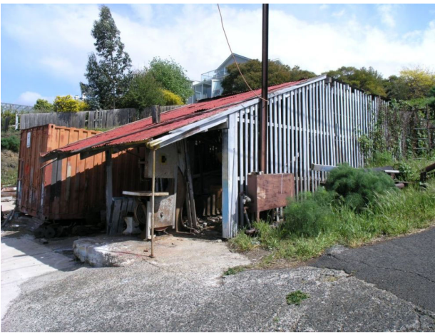
Image 30. Precinct F, B15 Engineering Shop
