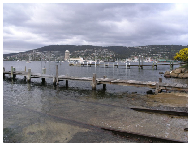
Image 32. View (V5) along the foreshore showing slips and jetties
