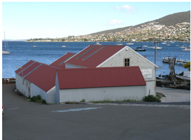
Image 27. Precinct F showing B13 Taylor Bros Storage Shed B14 Taylor Bros Workshops
