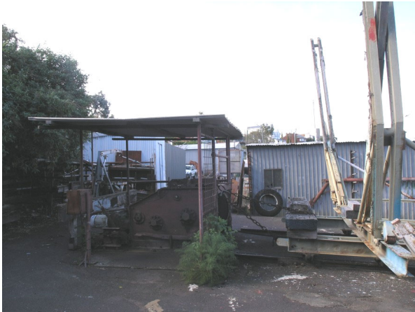
Image 22. Precinct E, B9 Winch and Shelter at the end of Muirs Slip
