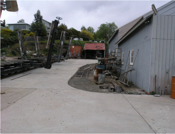
Image 28. Precinct F, Taylor Bros Slip and B14 Taylor Bros Workshop to the right
