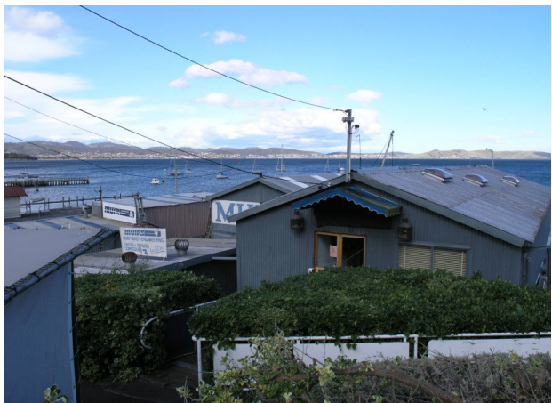
Image 25. View of B12 Muirs Workshops from embankment behind
