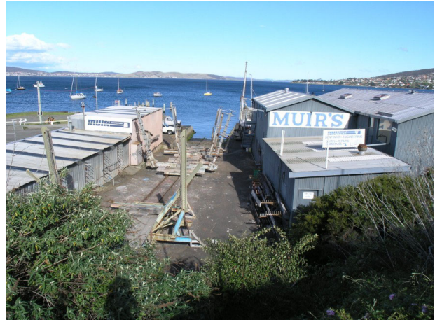
Image 23. View (V2) of Precinct E from embankment behind, B11 and B12 on the right and B8 on the left side with Muirs slip in between
