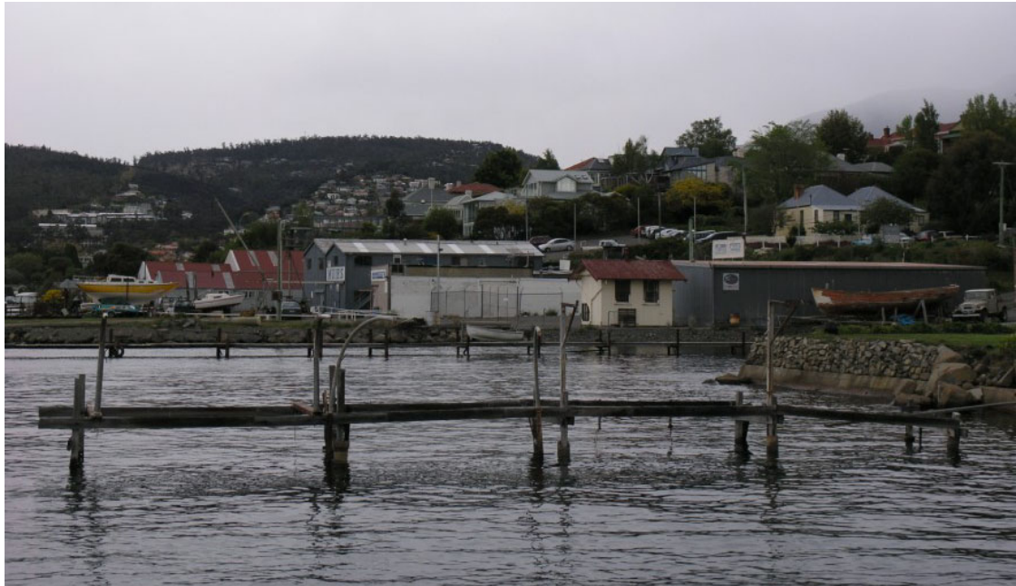
Image 5. View (V4) from Purdon and Featherstone jetty towards the Battery Point Slipyards showing the industrial landscape of groupings of buildings and jetties for each slip site and the Mariners Cottage (B10) on the ridge.
