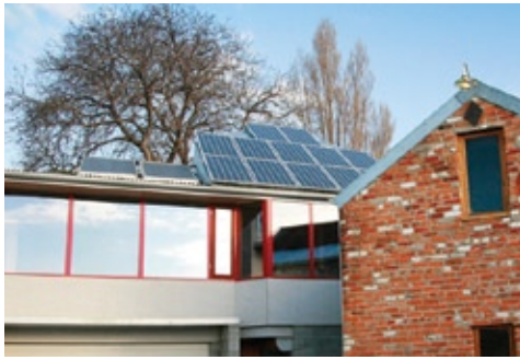
Fig. 10 Solar collectors at the Sustainable House Macquarie Street (a) north facing double glazed low-e windows for space heating (b) flat plate collectors for hot water, and (c) photovoltaic collectors for electricity.
