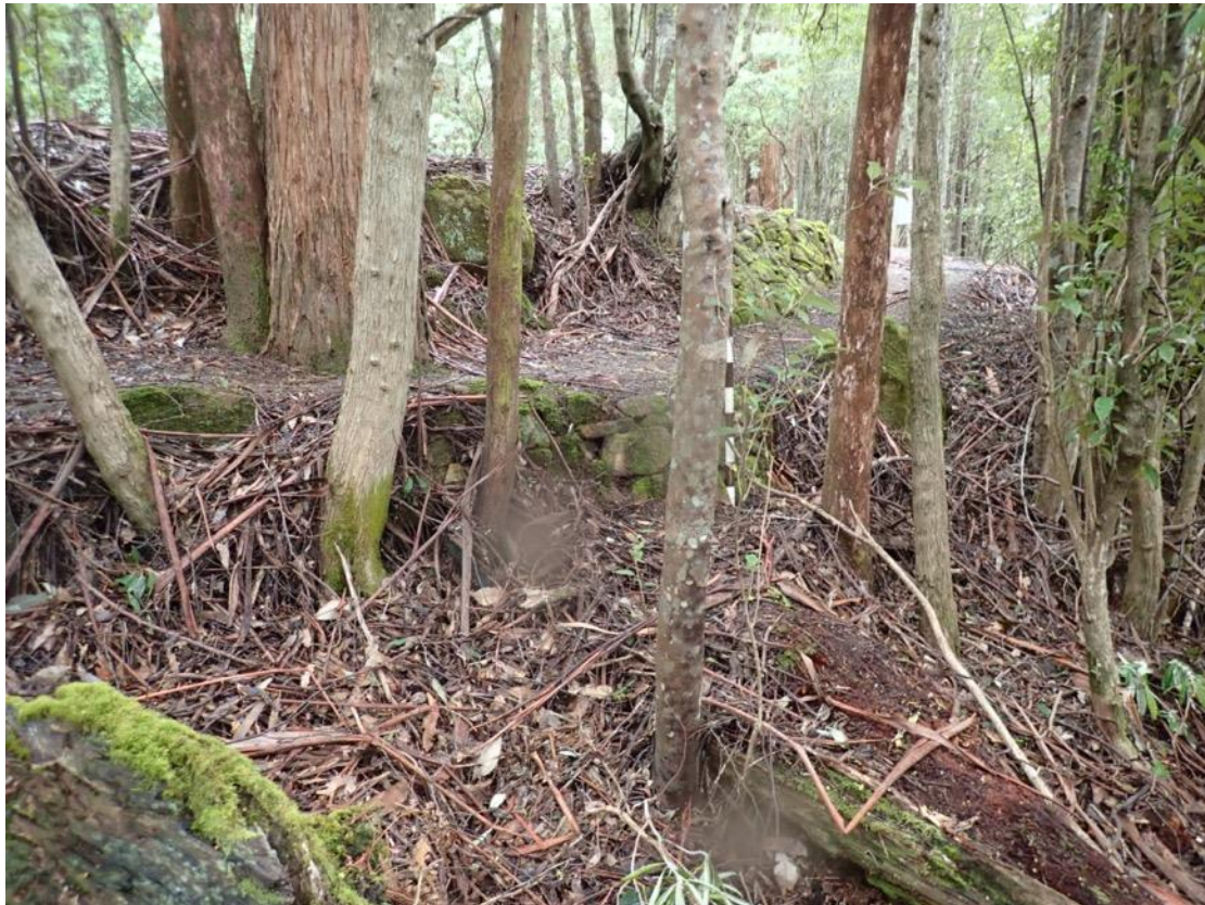
Figure B.1.1 View west showing the entrance to the Circle Track adjacent to Pinnacle Road. Shown in the centre of the photograph is the random coursed rubble supporting structure below the track. The scale has 100mm marks.
