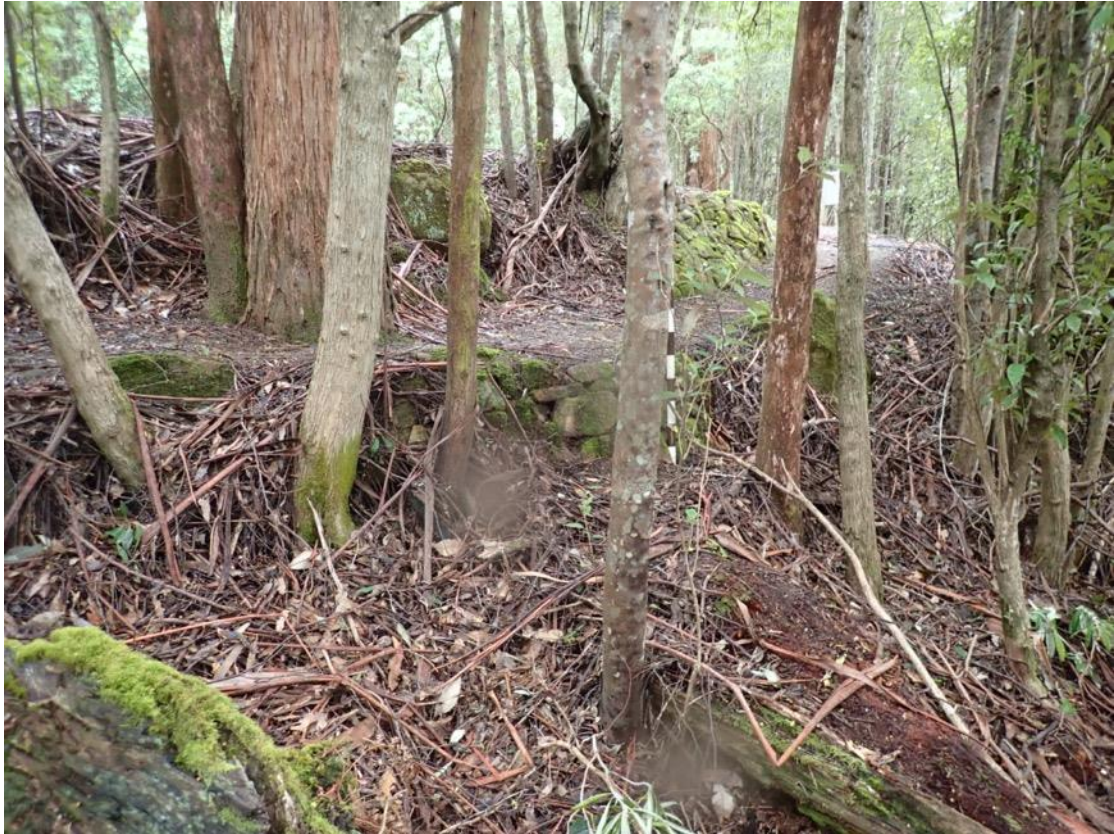
Figure 5.2.1 View west showing the entrance to the Circle Track adjacent to Pinnacle Road. Shown in the centre of the photograph is the random coursed rubble supporting structure below the track. The scale has 100mm marks.
