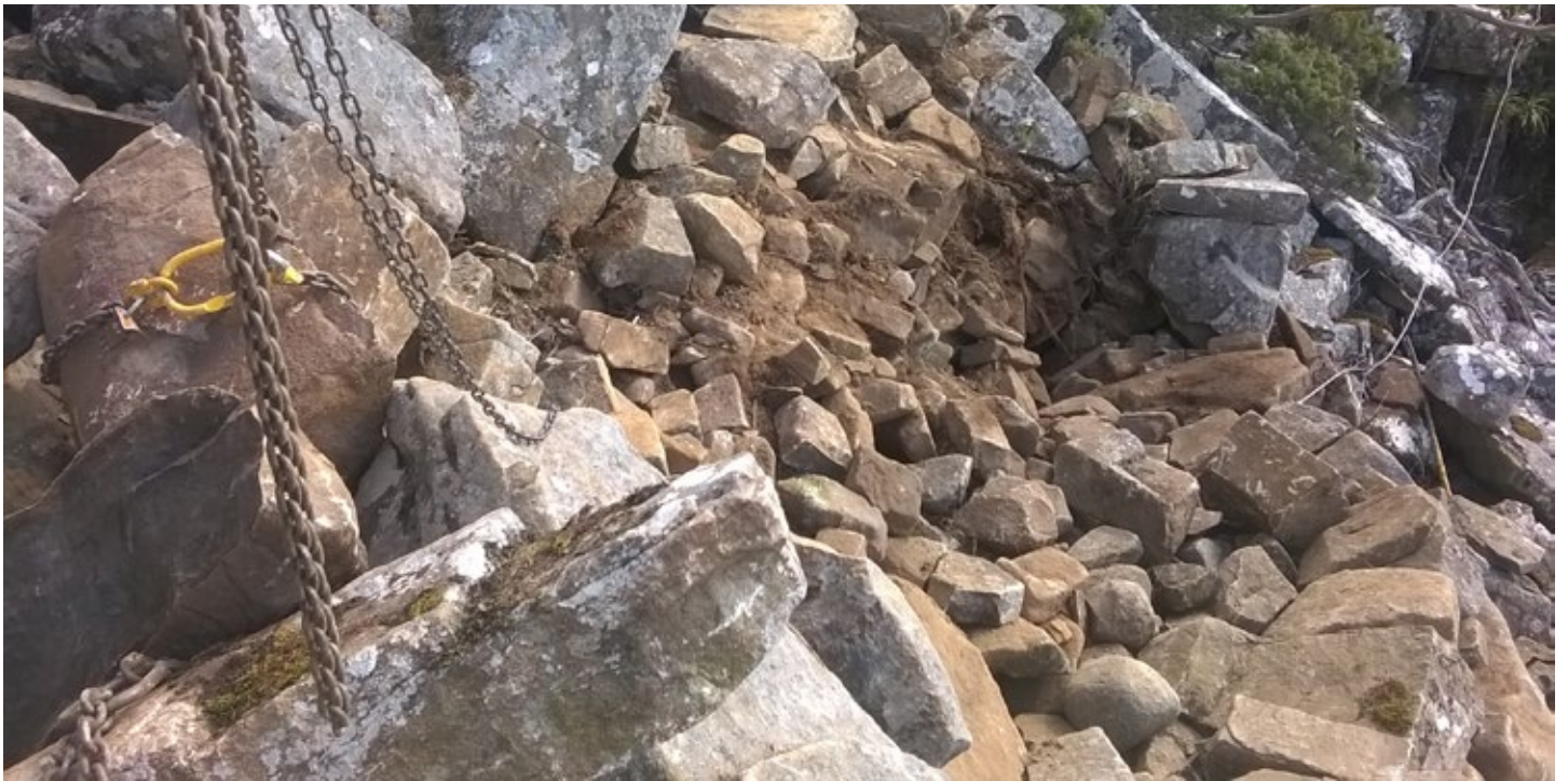
Winching boulders into place
